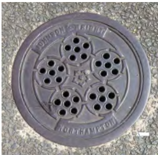
Picture 4 Johnson & Wright coal-hole cover over domestic, sub-pavement storage in Watkin Terrace
