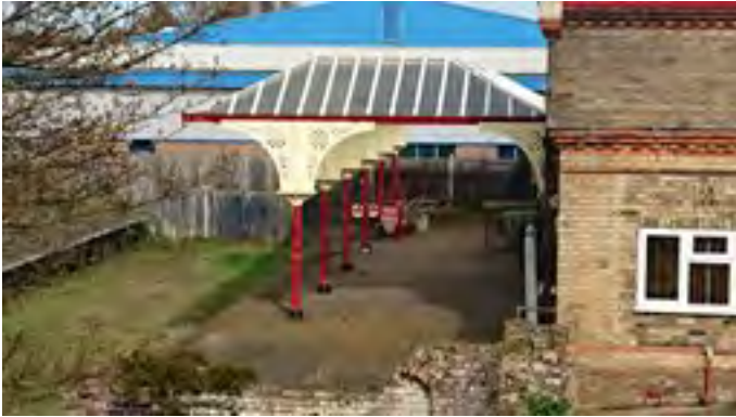
Barwell ironwork at former Potton station, Bedfordshire
